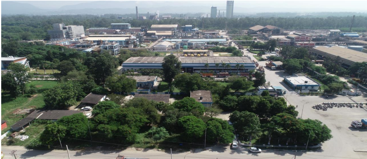
Manufacturing units: Location: Ropar, Punjab (India)
