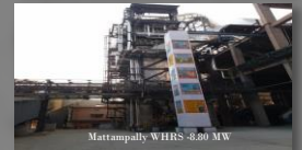
Mattampally WHRS -8.80 MW
