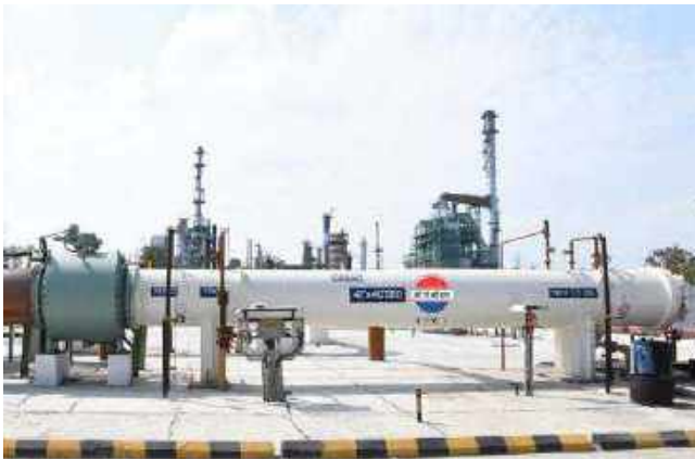
New 42" crude oil pipe line
