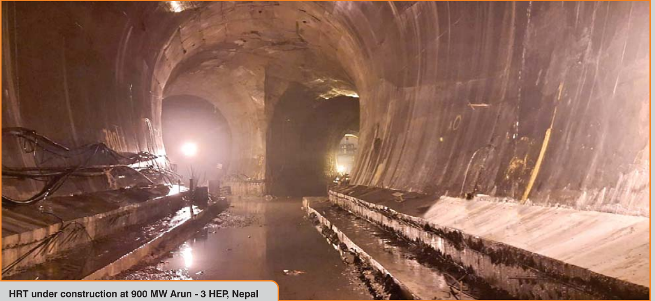
HRT under construction at 900 MW Arun - 3 HEP, Nepal
