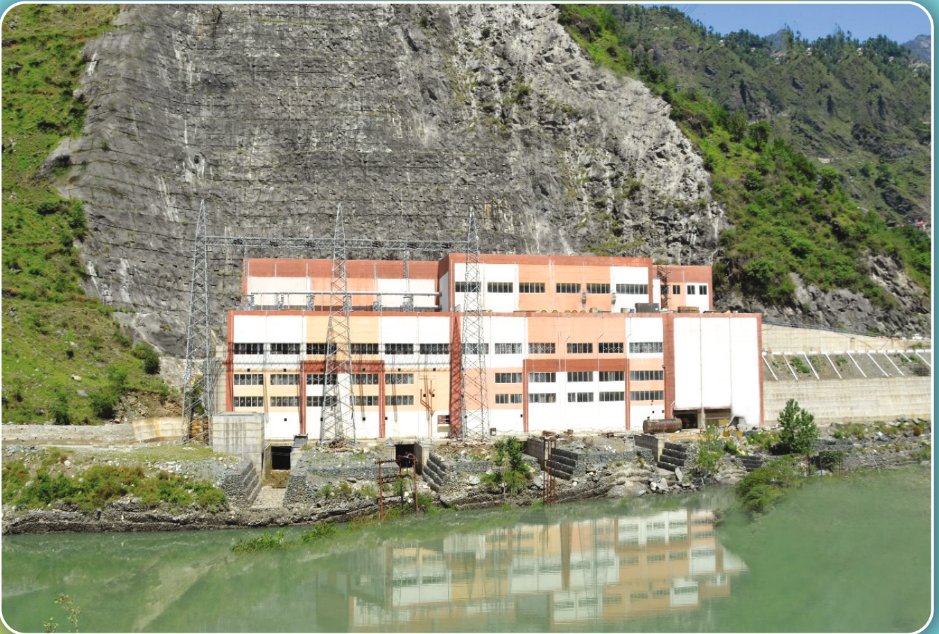
800 MW Parbati-II Project (Himachal Pradesh) - Surface Power House
