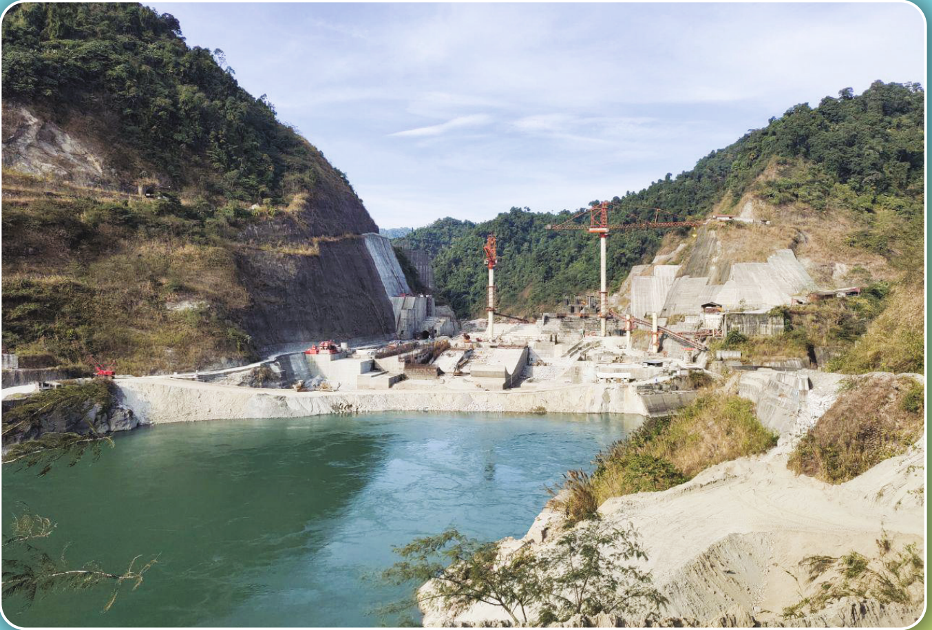
2000 MW Subansiri Lower Project (Arunachal Pradesh/ Assam) - Dam under construction
