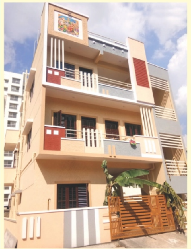
G+2 Work Hegde Nagar
