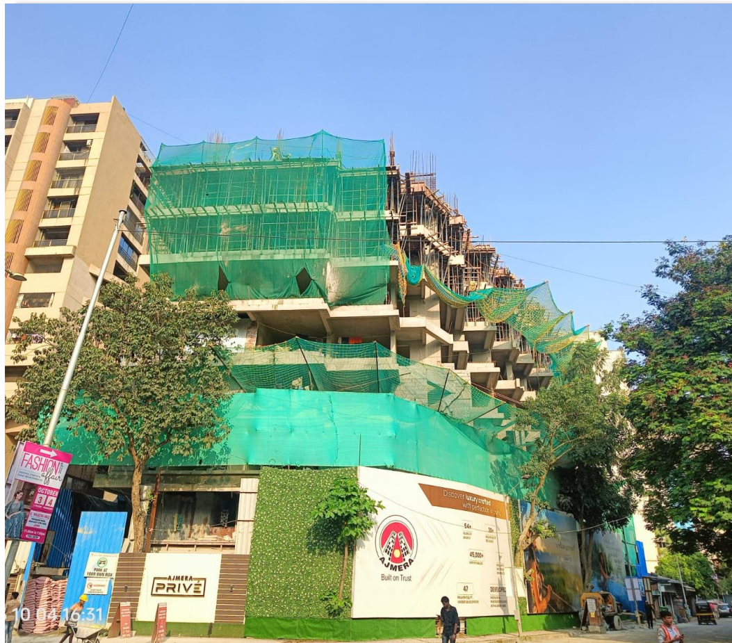
8th Floor Slab WIP
