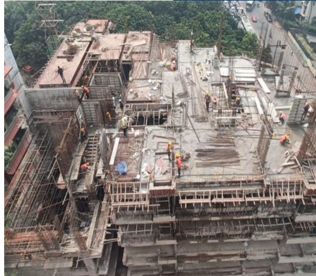
Reinforcement Work in Progress
