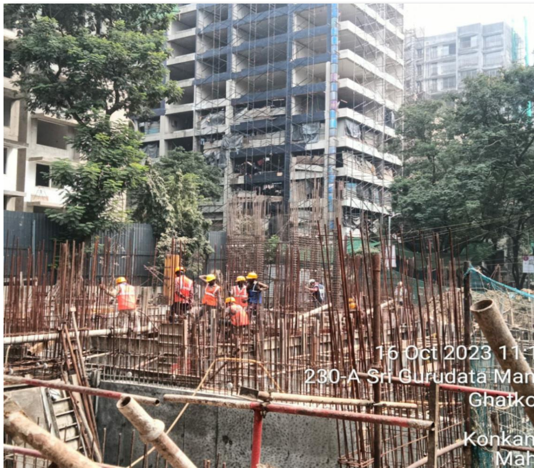
Concreting of Parking WIP
