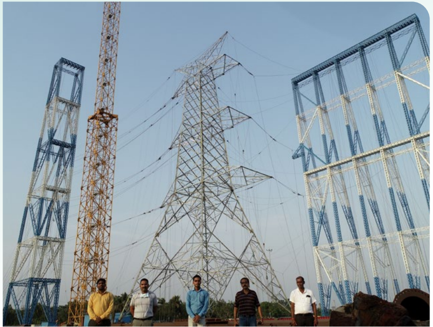
765kV Transmission Tower
