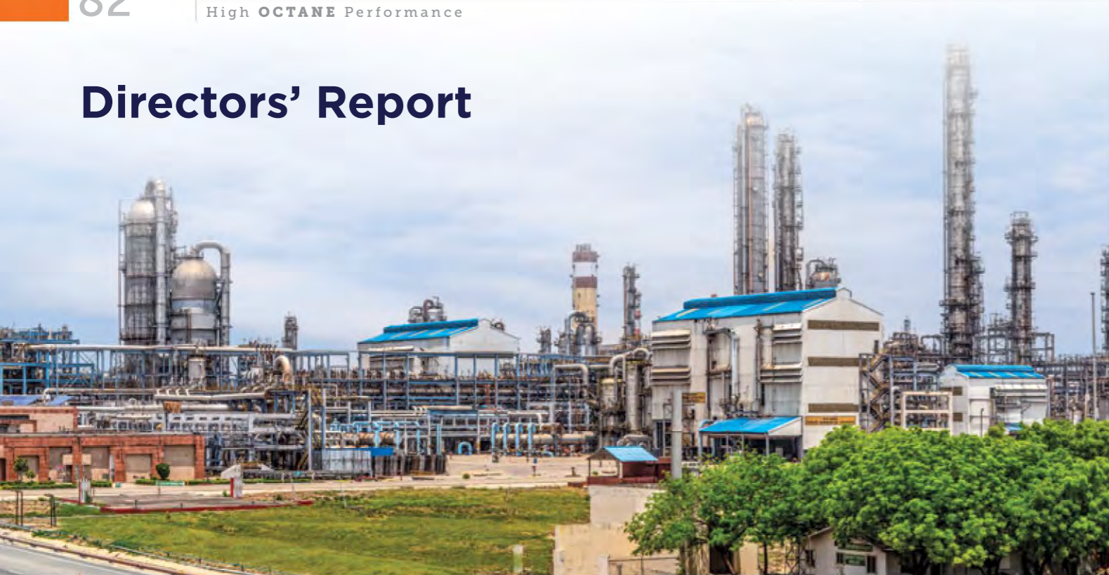
A panoramic view of IndianOil's Panipat Refinery
