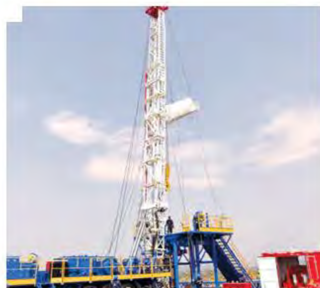
Aakash-XIV Rig carrying out well completion operation at well no. BK-51 well in the Coal Bed Methane (CBM) Block BK-CBM-2001/1 located in Bokaro, Jharkhand
