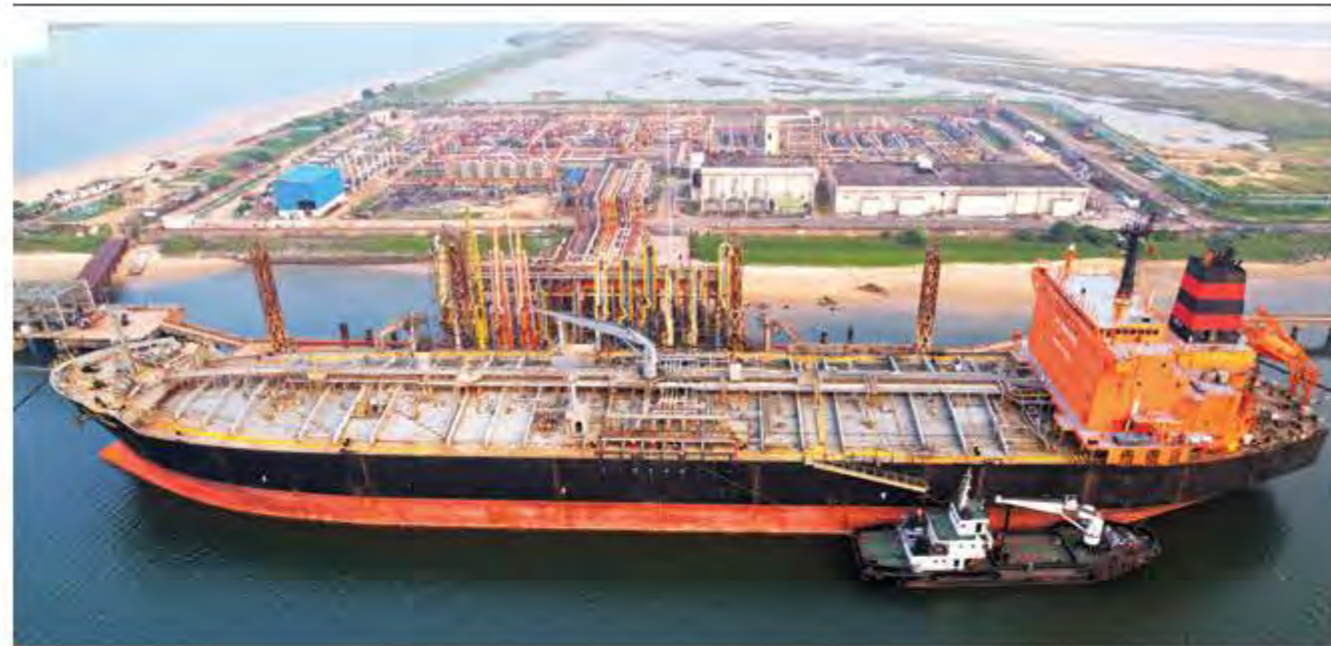
IndianOil Petroleum Product handling through tankers in South Oil Jetty at Paradip Port
