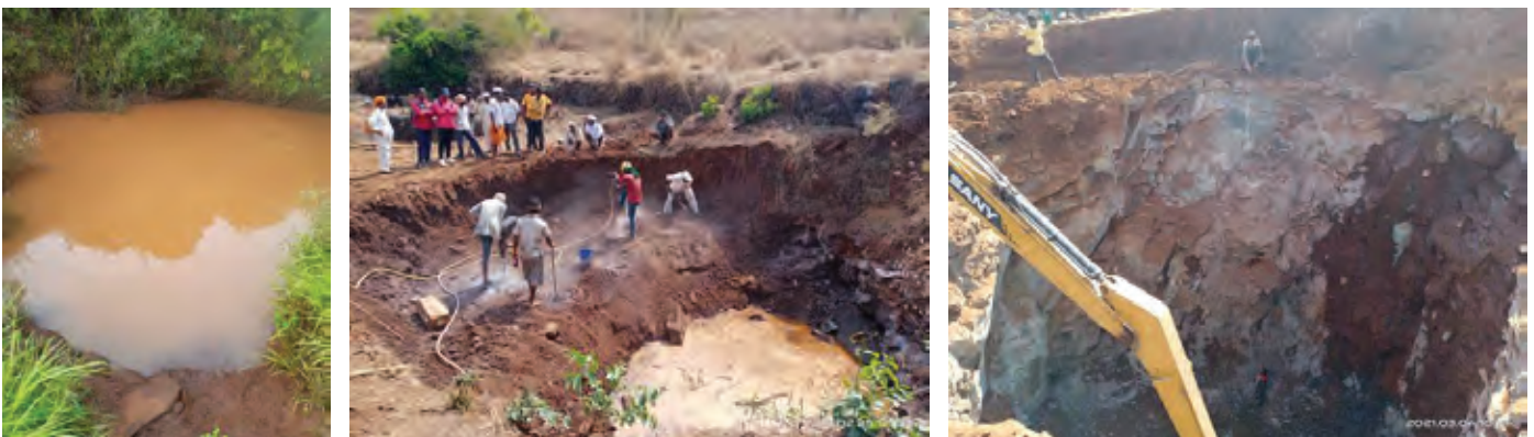
Figure 6: Well construction work-in-progress at Nigdicha Wada village
