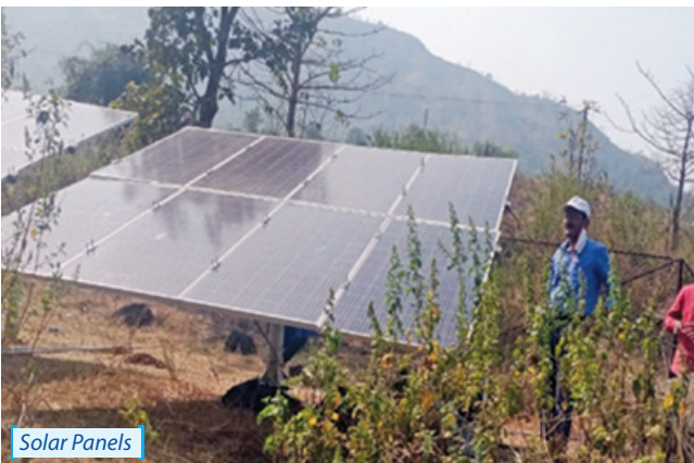
Inauguration of Solar Power
