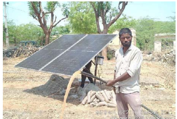
Installation of solar water pump sets that provide water for animals in Ranakpur Wildlife Sanctuary, Rajasthan.
