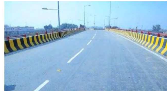
Construction of 2 lanes at Sonapat
