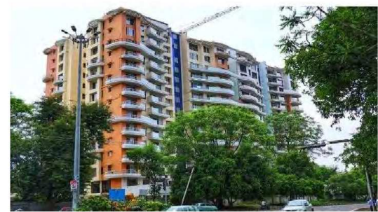
Construction of 96 flats at Tulsi Tower, Bhopal
