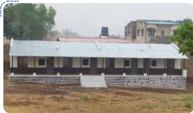
New Ashramshala school building ready in Mokhada
