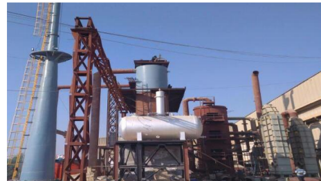
Kisan Phosphates, Haryana: Fertilisers Plant
