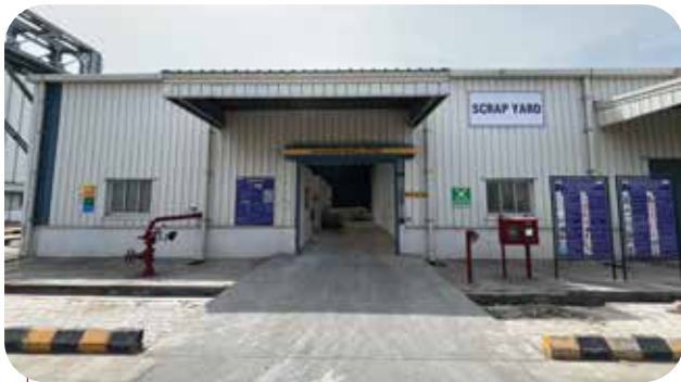
Dedicated Scrapyard Facility for Hazardous Waste Storage
