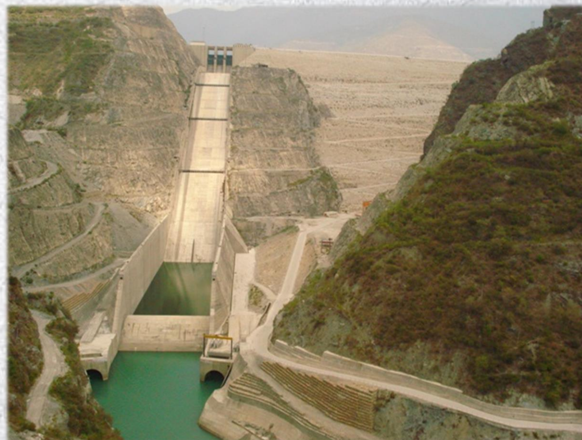
Tehri Dam, Garhwal
