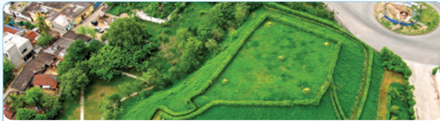
Dalma View Point, Jamshedpur. Municipal solid waste dump transformed into a lush green picnic area
