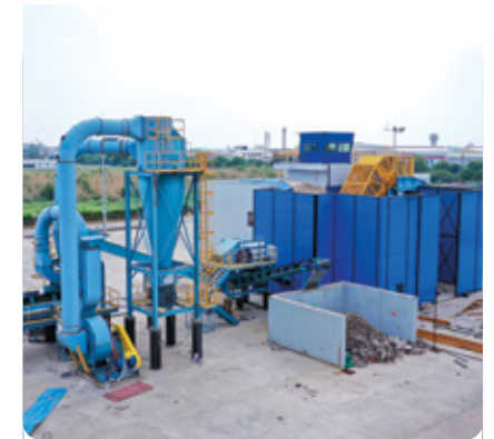
Steel Recycling Plant, Rohtak
