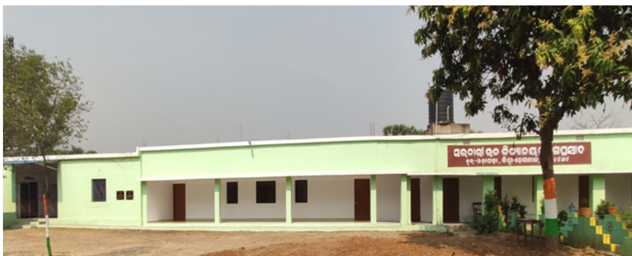
Construction and renovation of classrooms at Government High School, Kharagprasad, Odisha
