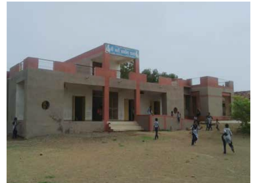
BEAUTIFICATION OF KHAREDI SCHOOL USING SPECIAL PAINT
