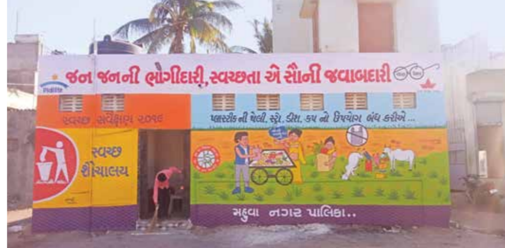
RENOVATION OF COMMUNITY TOILETS IN MAHUVA
