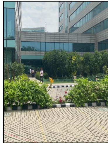
View of Tower 5
