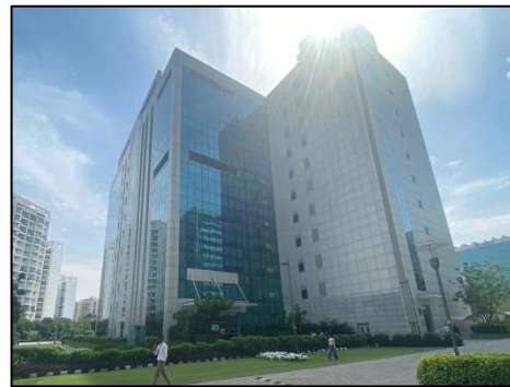
External View of Subject Property
