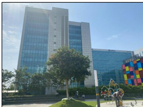
External View of Subject Property
