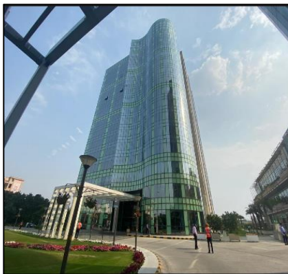
View of Block 5
