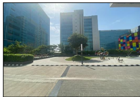
External View of Subject Property
