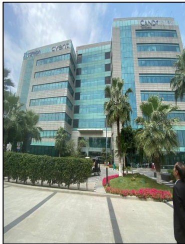
View of Tower 3 A & B
