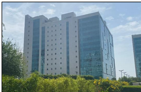
External View of Subject Property
