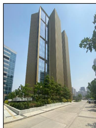
View of Tower 11
