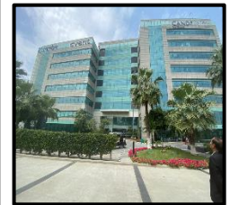
Tower 3A & B of Subject Property
