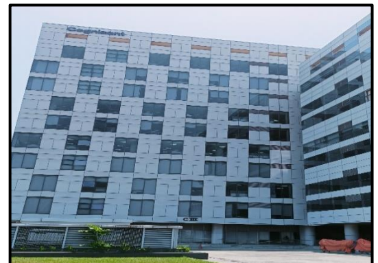
View of Tower C3
