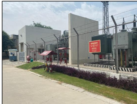
View of HSD yard
