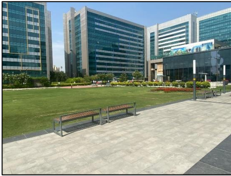
External View of Subject Property
