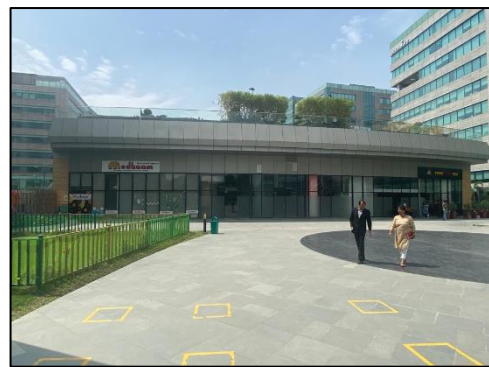
View of Amenity Block (Tower 4a)
