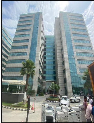
View of Tower 1 A & B
