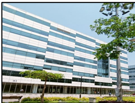
View of Tower G1
