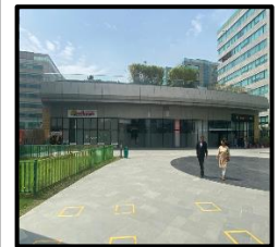
Amenity Block (Tower 4A) of Subject Property
