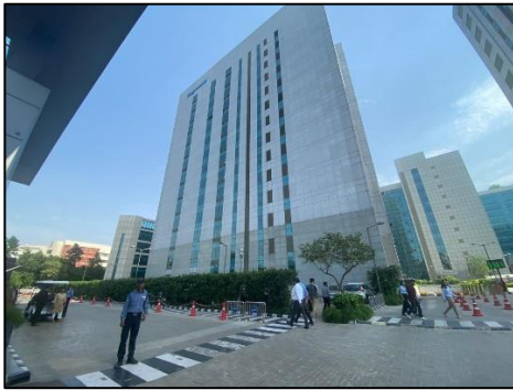
External View of Subject Property
