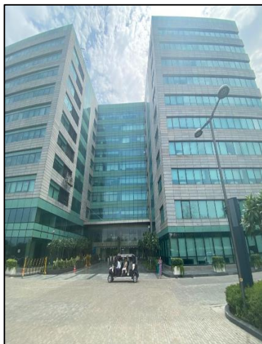
View of Tower 6 A & B
