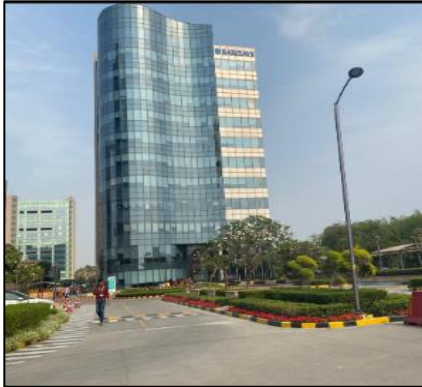
View of Block 1
