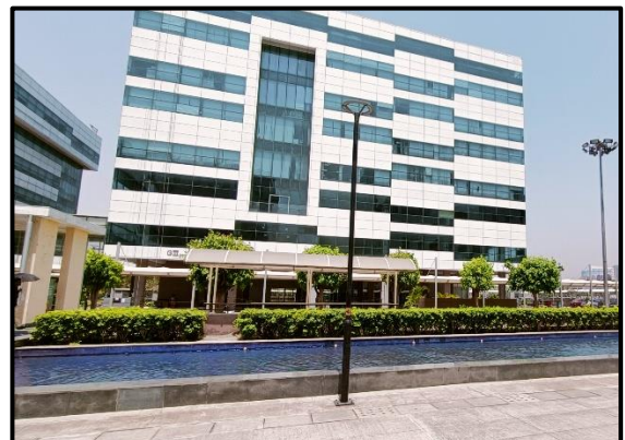
View of Tower G3
