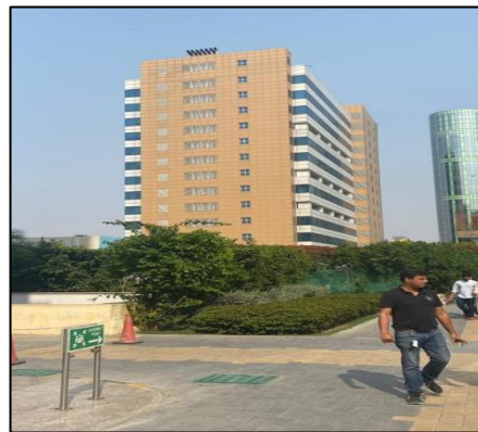
View of Block 6
