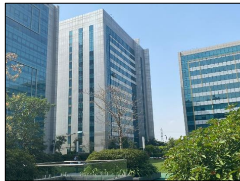
External View of Subject Property
