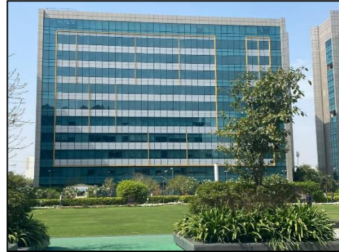
External View of Subject Property
