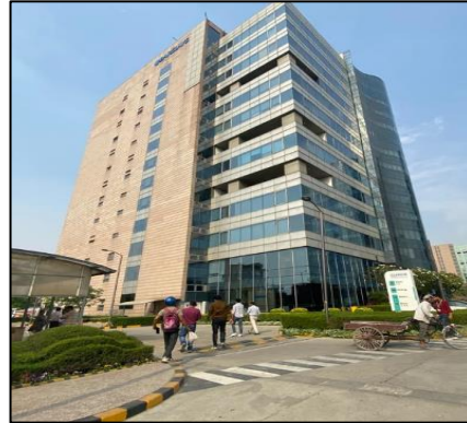
View of Block 2
