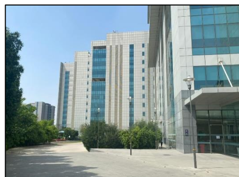
External View of Subject Property
