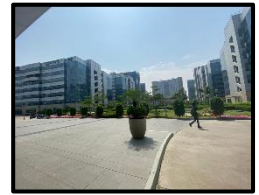
External View of Subject Property
