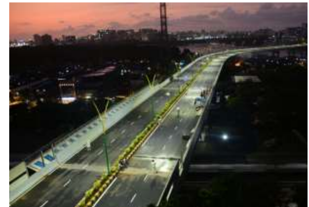
BKC- Chunabhatti Flyover
