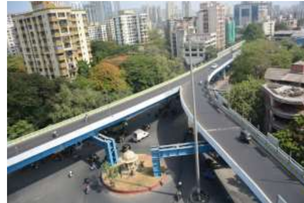
Meenatai Thakre Flyover
