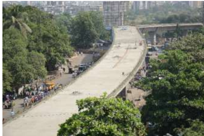
Kalwa Bridge Thane
