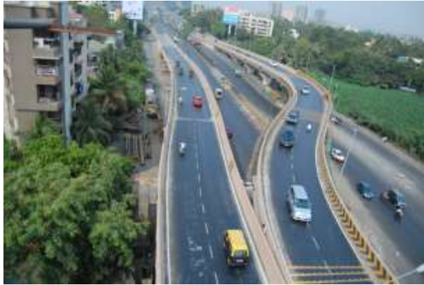
Amar Mahal Flyover
