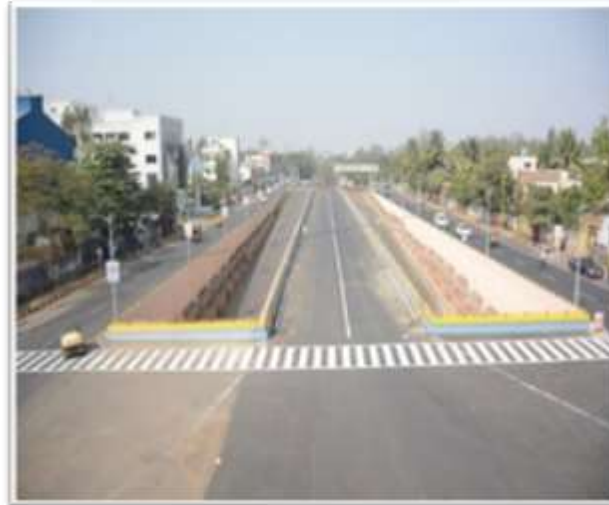
KSB Underpass, Pune
