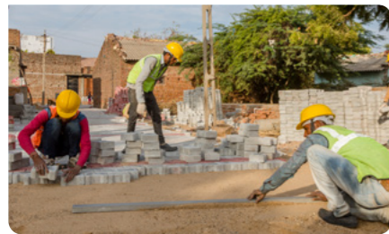
Paved street laid in one of the project village
