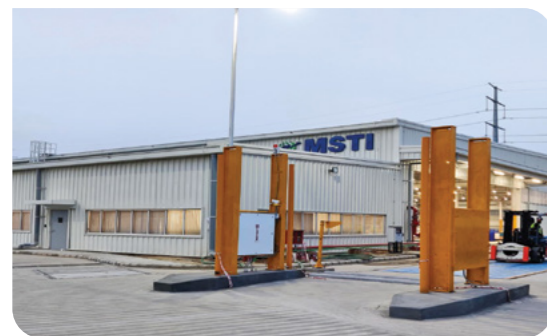
A view of MSTI facility
