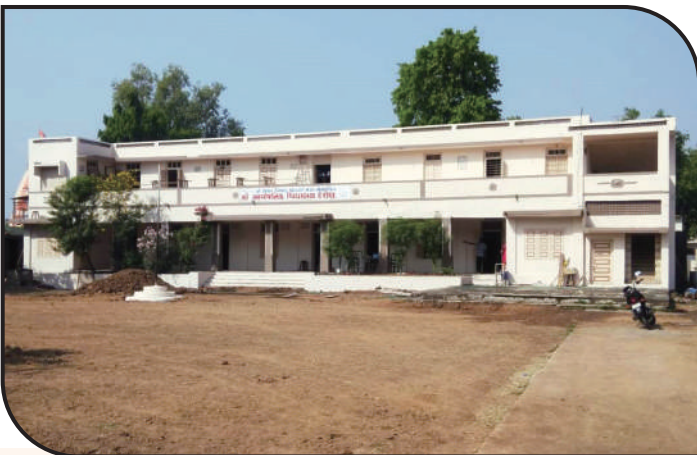
Renovation of School Building - Village: Derol, Dist: Bharuch.
