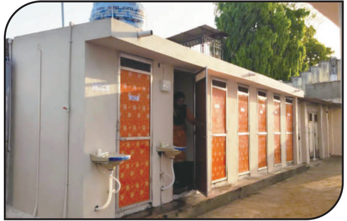
Construction of Toilets for Dandi Marchers - Village: Derol, Dist: Bharuch.
