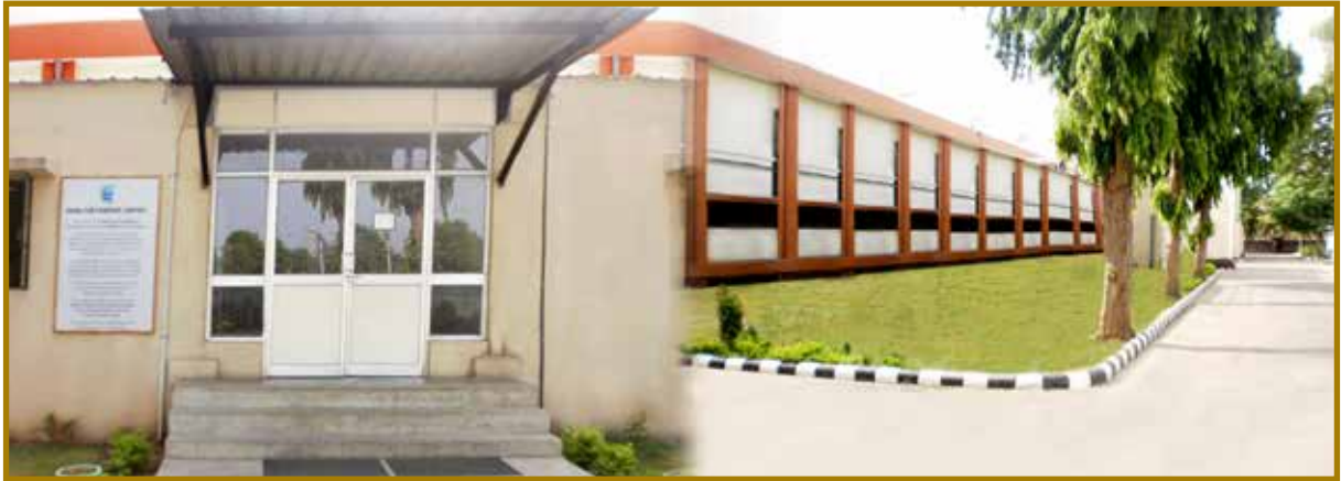
Kanjari Factory - Gujarat
