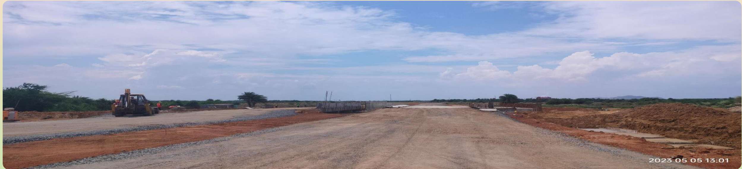
TSSEL- Access road & bridge over water body
