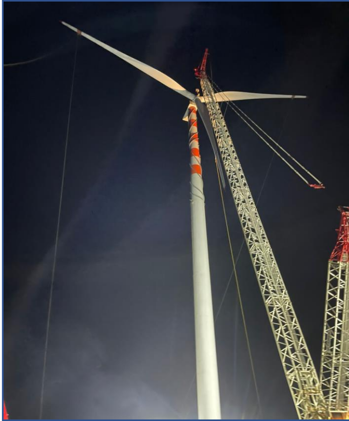
WTG Erection work in progress
