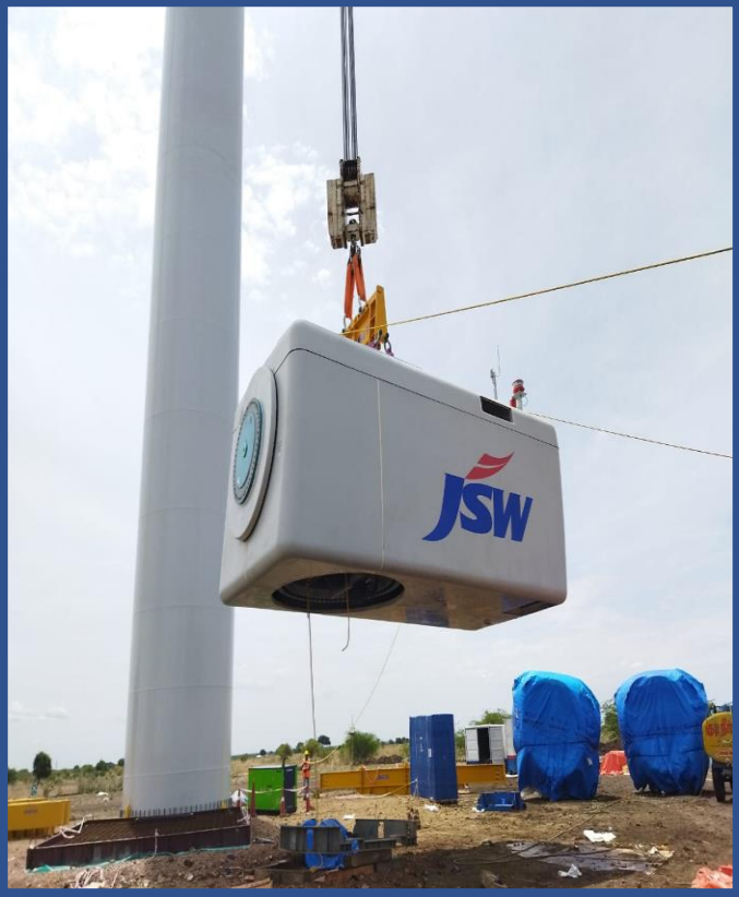
Nacelle Erection work in progress
