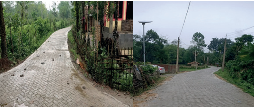
Constructed road in the Margherita region of Assam
