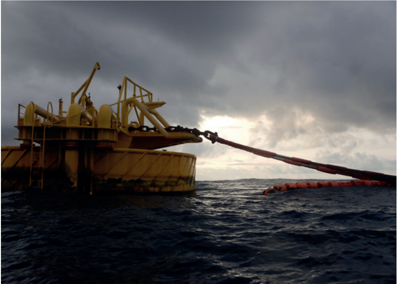
B-80: Post Installation of Single Point Mooring system (SPM)
