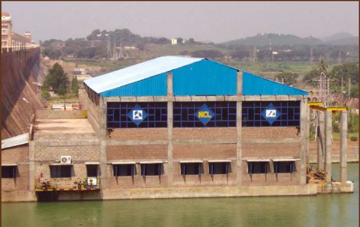
Hydel Power House at Tungabhadra Dam.
