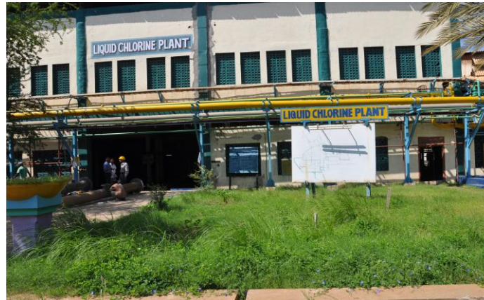
Liquid Chlorine Plant
