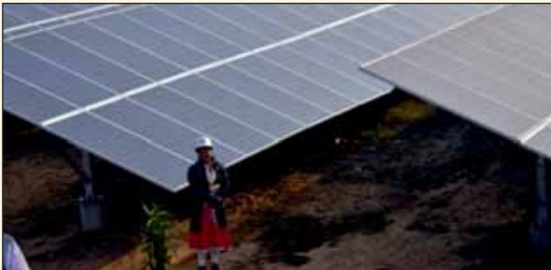
Solar panels of the Power Plant at RSP.
