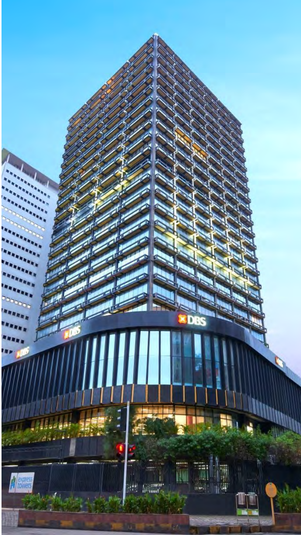
Express Towers Mumbai (0.5 msf)
