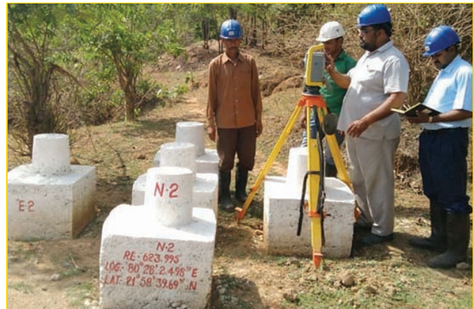
Monitoring of subsidence pillars by Total Station at Munsar Mine
