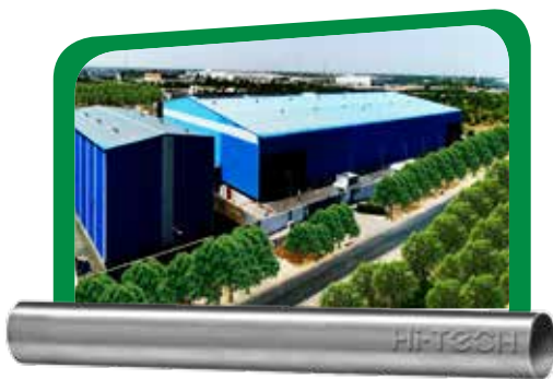
Sanand, Gujarat Installed capacity of 1,25,000 MTPA
