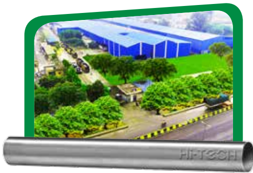
Sikandrabad, Uttar Pradesh (Unit-1) Installed capacity of 2,19,000 MTPA
