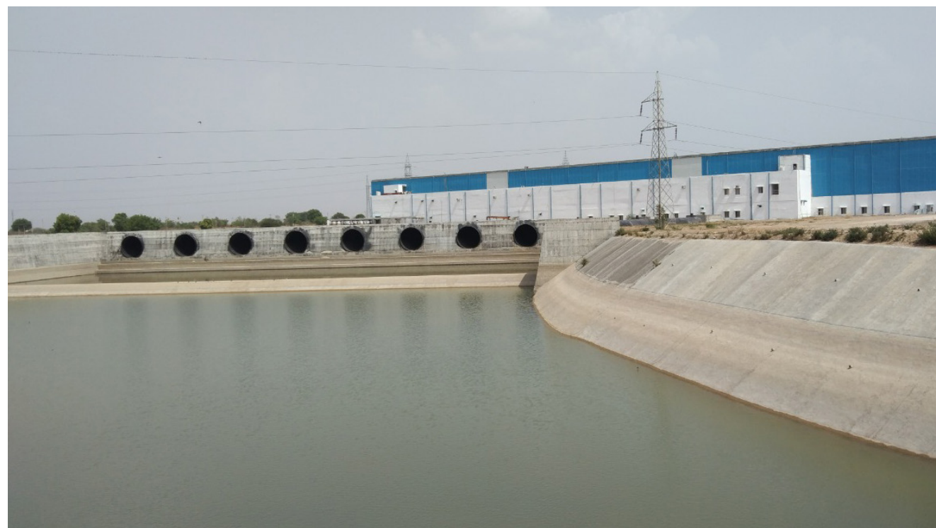
REC funded electro-mechanical and associated civil works at Indirama Flood Flow Canal Scheme in Telangana
