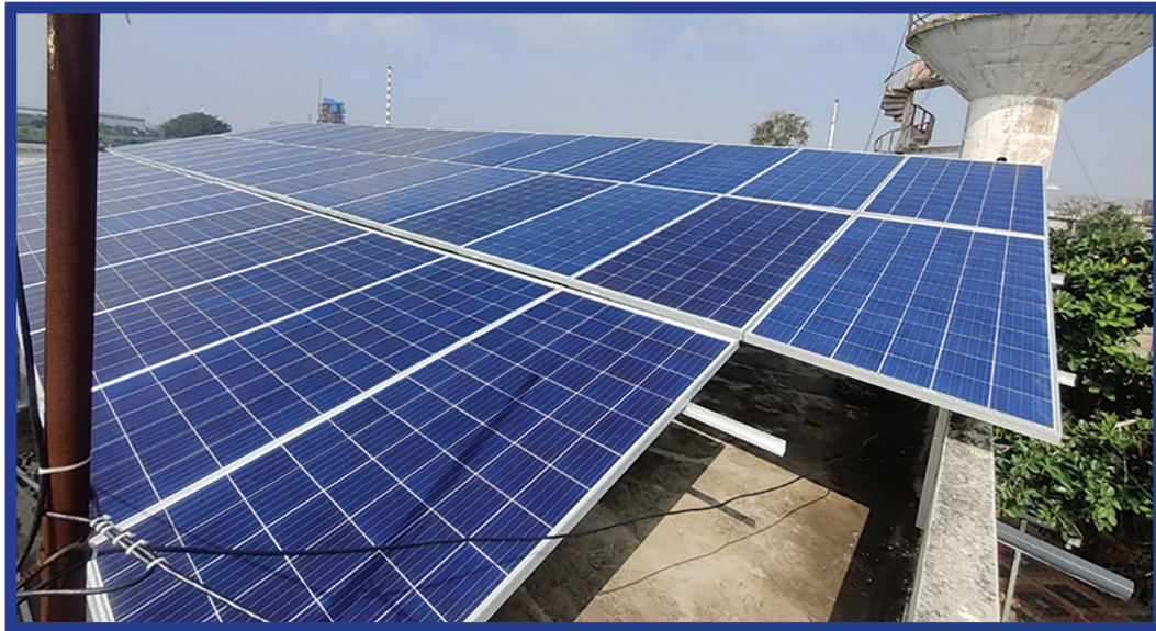
Installation of 25 KW solar panels at Grampanchayat office, Vadadla, Dahej
