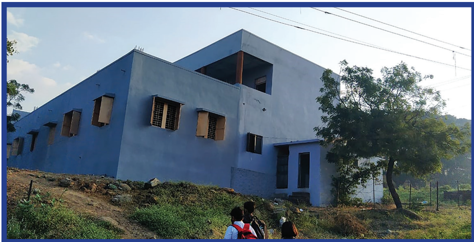
Construction of 3 classrooms for the Vocational Skill Training Centre, Kurkumbh
