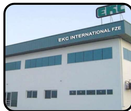
Plant II – Dubai
