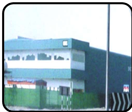
Plant I – Dubai
