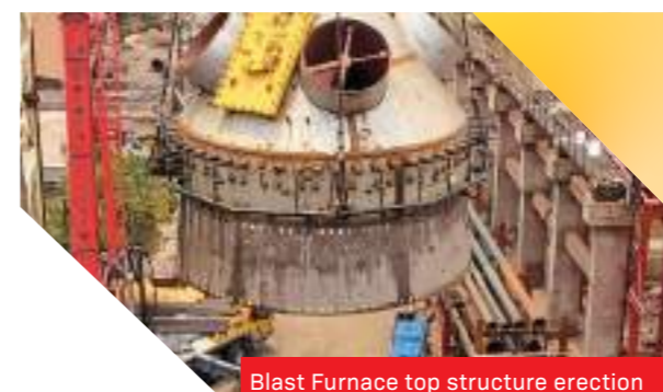
Blast Furnace top structure erection
