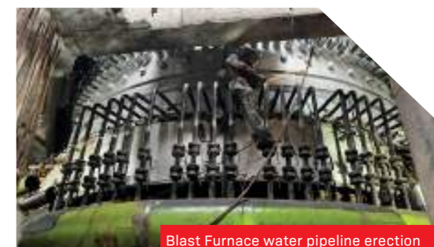
Blast Furnace water pipeline erection
