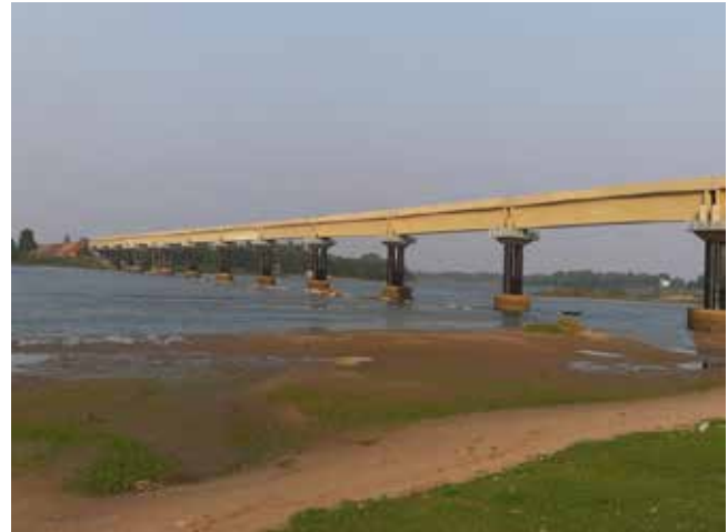
Bridge No. 134 (22x43.8m PSC girder) over River Mahanadi, Odisha
