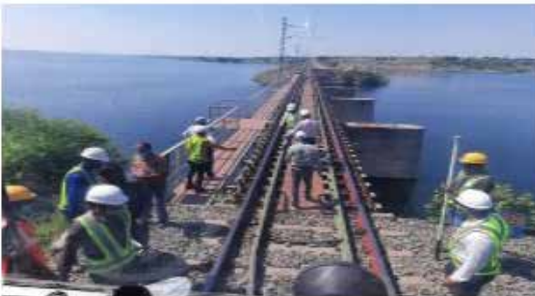
Commissioning of doubling of rail line between Kulali - Savalgi section on 11.11.2020
