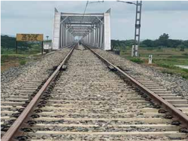
Bridge No. 133 (5 x 45.7m Steel Girder)
