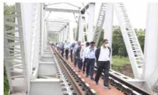
CRS Inspection of Bhimalgondi-Bhandarkund section on 22.08.2020
