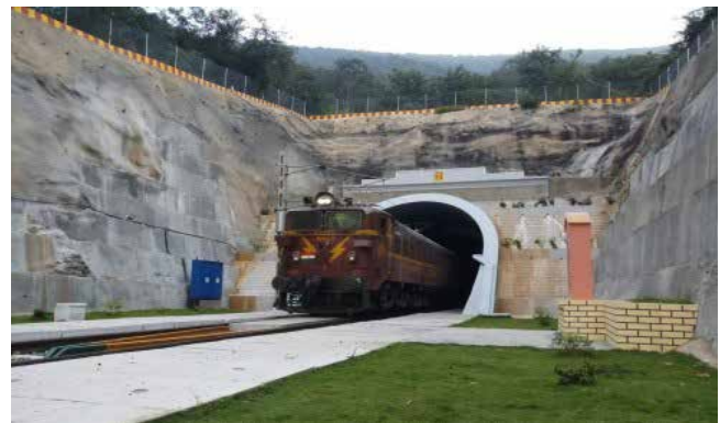
6.7 Km long tunnel
