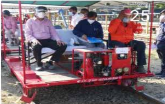
Commissioning of 3rd Railway line between Habibganj-Bhopal
