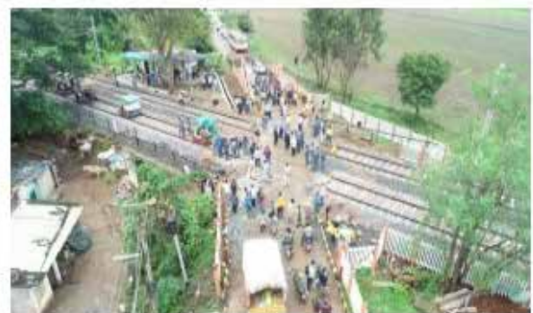
Commissioning of Unkal-Dharwad doubling project on 19.10.2020
