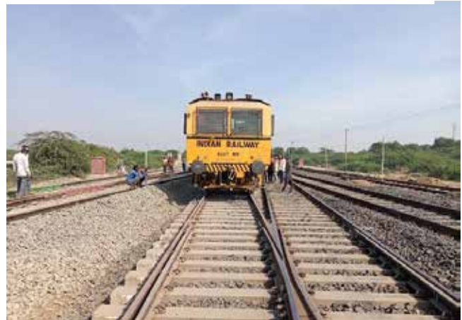
Execution of Doubling work
