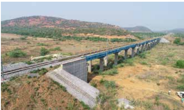
Major Bridge (14 x 18.30 M PSC Girder)
