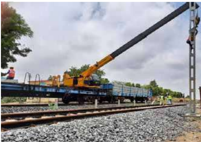
Execution of Railway Electrification work
