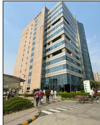
View of Block 2
