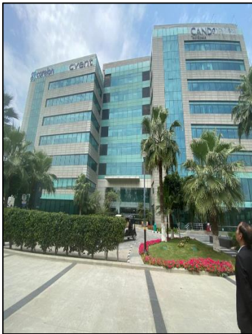
View of Tower 3 A & B
