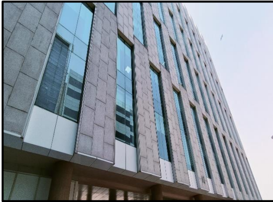
View of Tower A1
