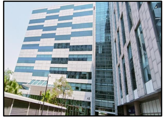
View of Tower A3
