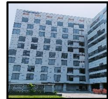
Tower C3 of Subject Property
