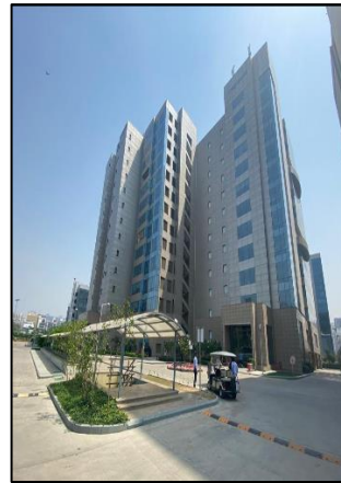
View of Tower 2
