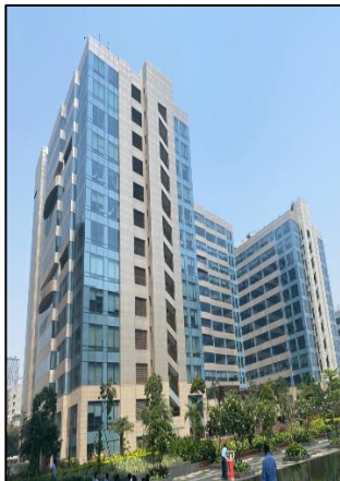
View of Tower 8,9,10
