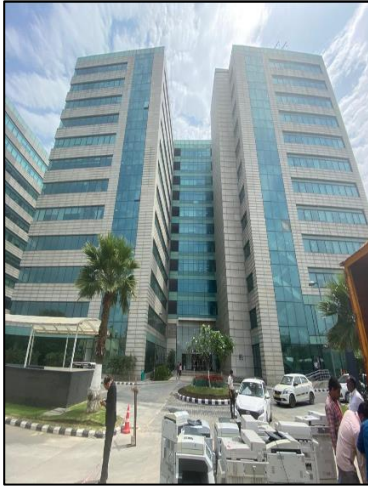
View of Tower 1 A & B
