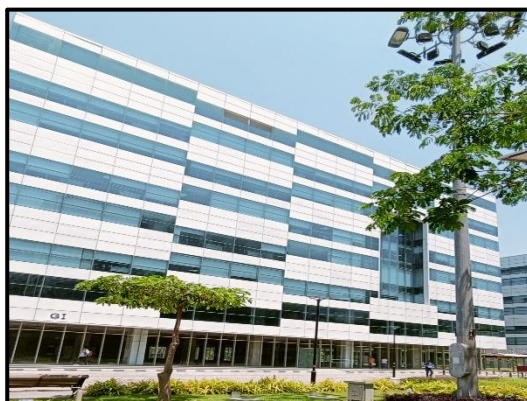
View of Tower G1
