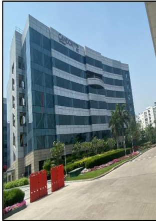
View of Tower 1
