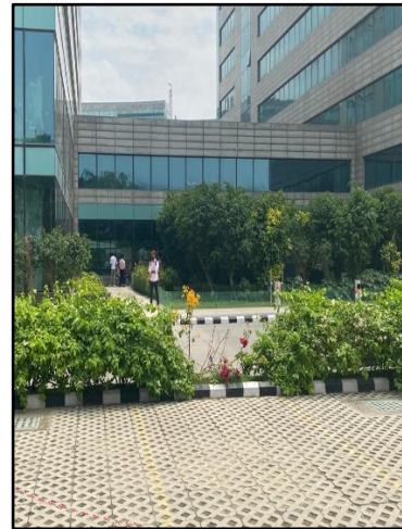
View of Tower 5
