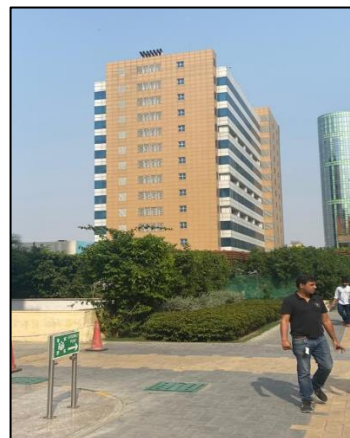
View of Block 6
