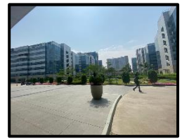
External View of Subject Property
