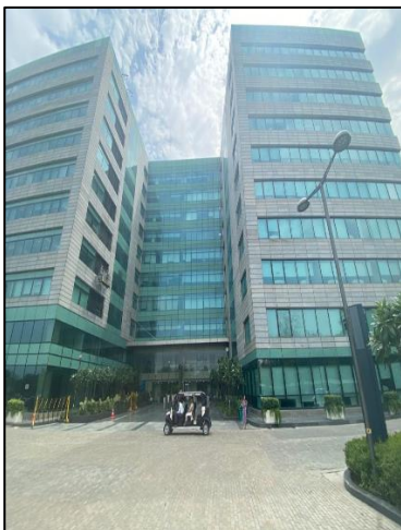
View of Tower 6 A & B
