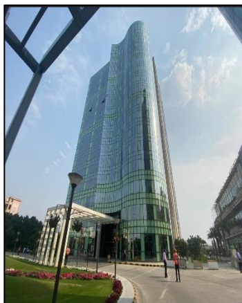
View of Block 5
