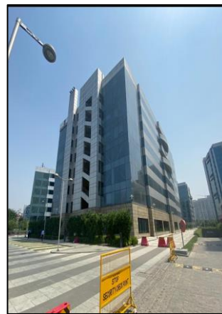
View of Tower 10
