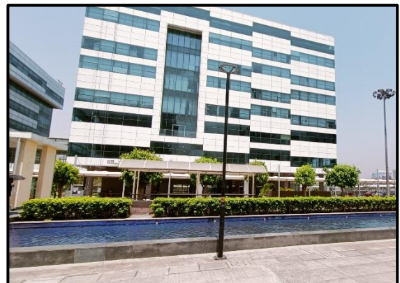
View of Tower G3
