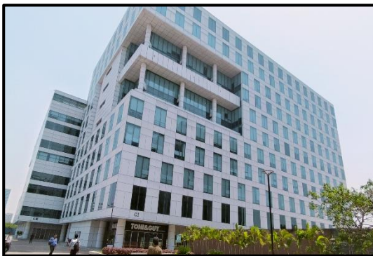
View of Tower C1
