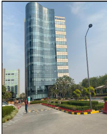
View of Block 1
