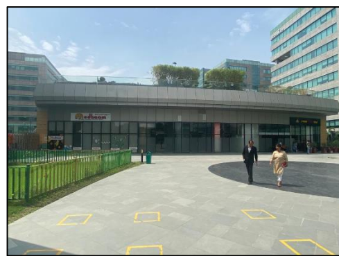
View of Amenity Block (Tower 4a)
