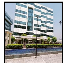
Tower G3 of Subject Property
