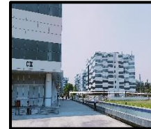
Tower G3 & C2 of Subject Property
