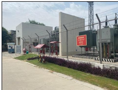
View of HSD yard
