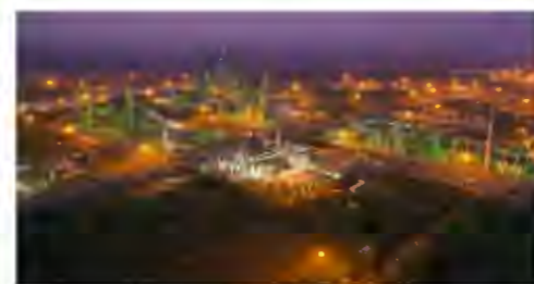
➤ BORL, BPCL's JV refinery inaugurated in Bina MP
