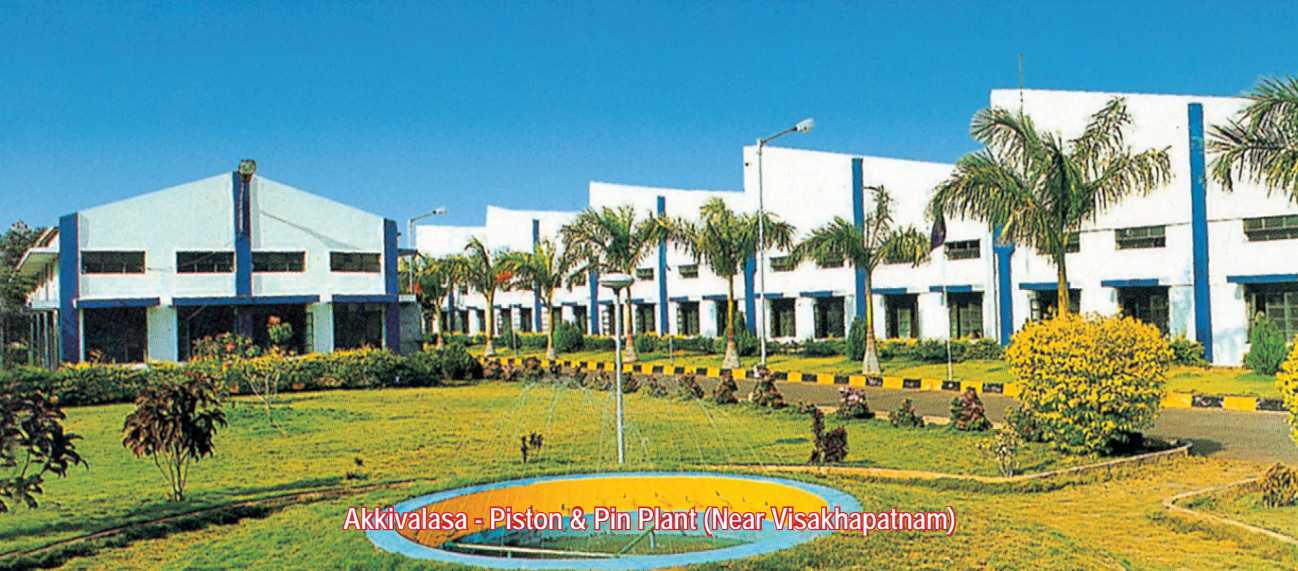
Varisam - Rings Plant (Near Visakhapatnam)
