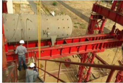
HP Heater Replacement 800 MW, CGPL Mundra 2
