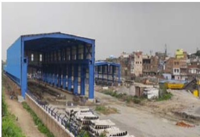
MEMU Shed at Kanpur-RVNL
