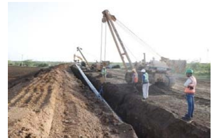
Lowering of Pipe Section, Mundra, Adani
