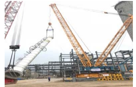
Urea Reactor Tank Installation At Ramagaundam, Telangana
