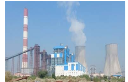
2x660 Mw STPS, Suratgrah - RRVUNL
