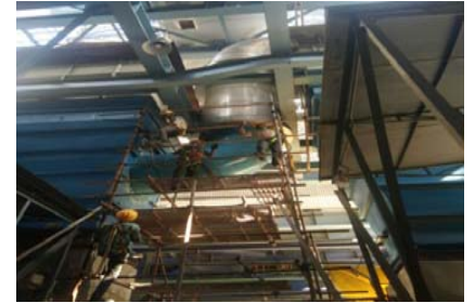
MSH Line Modification, 600 MW Singareni
