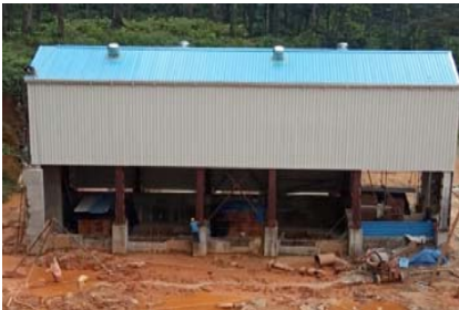
Implementation of Hydro Electric Project (2MW/5.14 Mu)-KSEB
