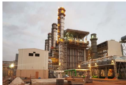
1,390 MW Waad Al Shamal ISCCPP, GE, KSA
