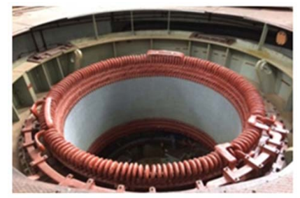
Implementation of Hydro Electric Project, 2 MW at Upper Kallar, KSEB
