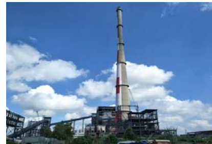
1x660 MW Harduaganj TPS, UPRVUNL
