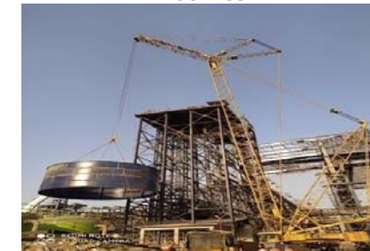
SMS II – Overhead Tank, Dolvi - JSW
