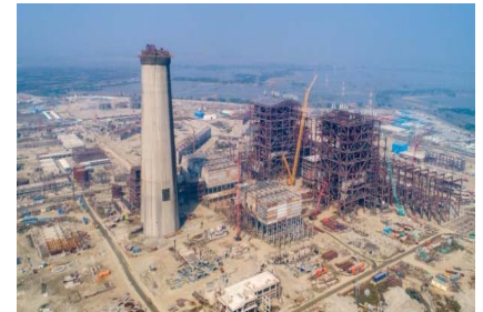
2X660 MW at Rampal, Maitree, Bangladesh-BIFPCL
