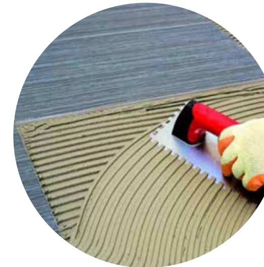
Tile and Stone Installations
