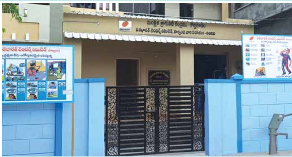
Safe drinking water plant at Kothagudem
