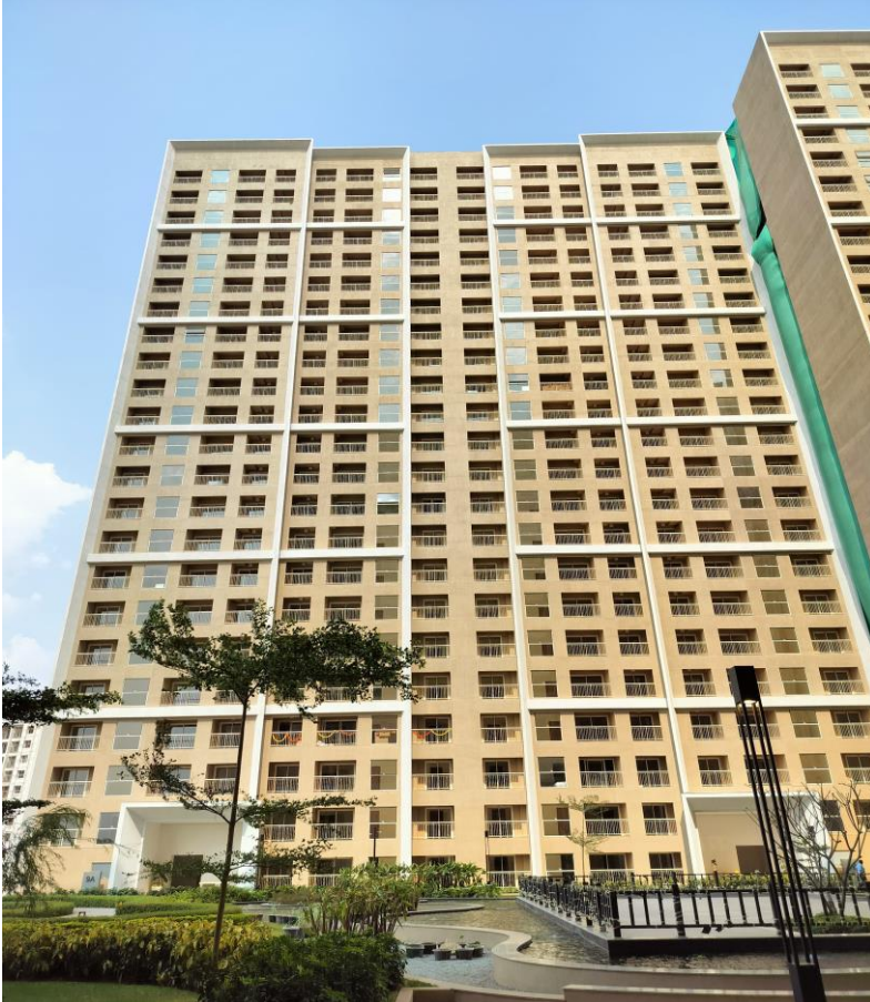
Wing 9A and 9B comprising of 2 tower G+23 floors Total SBA completed in Q4-FY24 – 182,591 sft (182 units)
