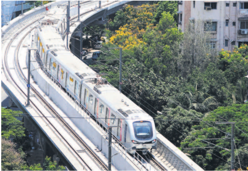
A host of Chinese companies have won contracts for ongoing infra projects in Mumbai city, including the Mumbai Metro.
