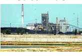
AHMEDABAD: As a pivotal component of the expansive barrage-cum-bridge project spanning the Sabarmati near the Torrent Powerhouse, the municipal authority is set to construct a rubber dam across the waterway. This project falls under the aegis of the Sabarmati Riverfront Development Corporation Limited (SRFDCL), which has initiated the tendering process for the initiative. Termed a rubber dam, also known as an air-filled rubber barrage, this structure will consist of a singular vulcanized rubber bladder system devoid of joints. This flexible system can be inflated or deflated according to the riverfront's water level and flow dynamics. The proposed rubber dam will extend over 30m and reach a height surpassing 2m. It will connect the Torrent power plant on the western bank to Camp Sadar Bazaar on the eastern bank.
