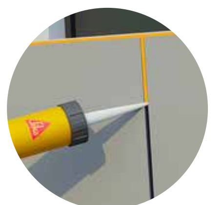
Facade gap filling
