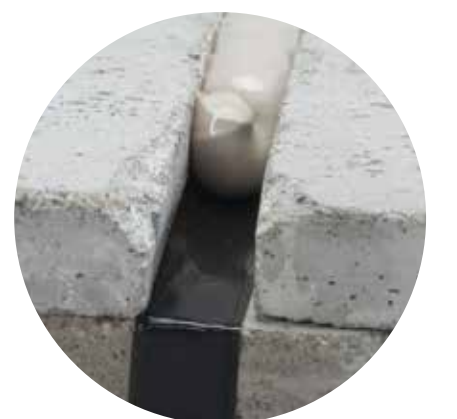
Construction joints gap filling
