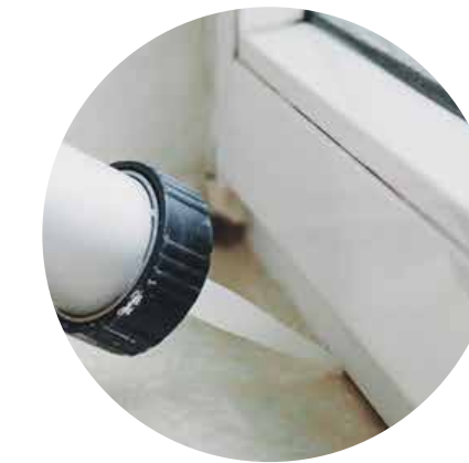
Doors and window gap filling
