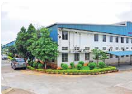
VISAKHAPATNAM (SEZ) Andhra Pradesh Product line: Ni-Cd batteries
